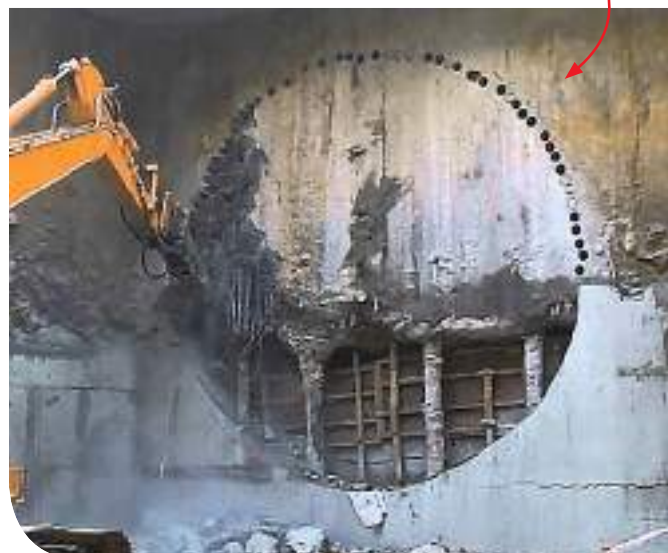
Removal of concrete and steel structure
